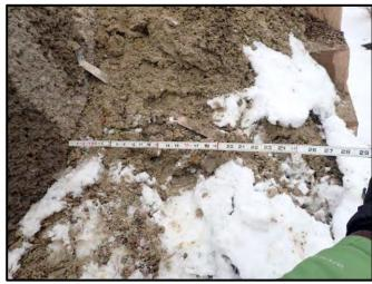
Figure 29: Collapsed area showed approximately 24 inches of backfilled space between walls
