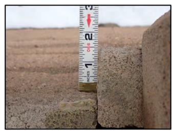
Figure 48: Displaced CMU fascia wall approximately 1.5 inches outward
