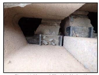
Figure 50: No gravel fill within block void
