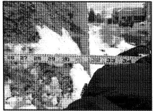
Figure 30: Lateral view attempting to align exterior face of CMU fascia wall with folding ruler
