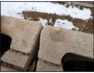
Figure 40: Adhesive on last course if block in Wall A to attach cap unit
