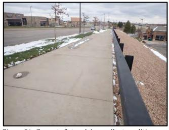
Figure 51: Concrete flatwork in excellent condition over retaining wall
