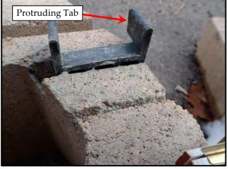
Figure 21: Closeup of plastic clip used to resist lateral loads with protruding tabs to set the batter of the wall
