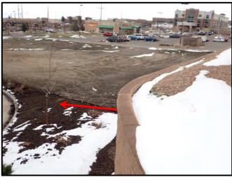
Figure 37: Outside radius of Wall A leans outward approximately 0.5°
