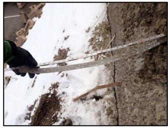
Figure 15: Straight wall tie with no evidence of bend from being turned down into the void of the CMUs
