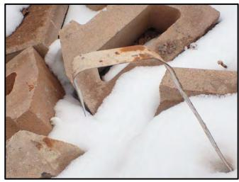
Figure 19: Sharp bend in wall tie where it was bent downward within void of CMU
