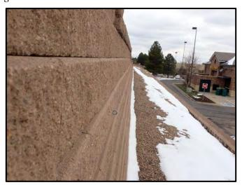
Figure 35: Wall B showing proper batter towards fill
