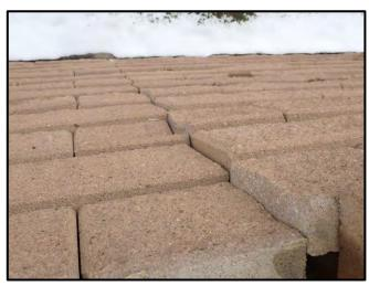
Figure 47: Second view of displaced CMU fascia wall showing the displacement is greater at the top
