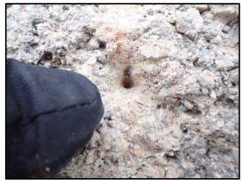
Figure 23: Void where PAF pulled out of shotcrete face of the soil nail wall
