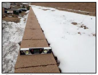
Figure 41: Wall A cap unit leaning outward at 2.2°
