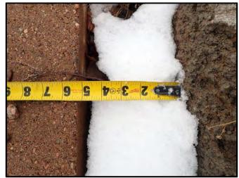
Figure 24: Space between shotcrete wall and back of cap unit approximately 5 inches
