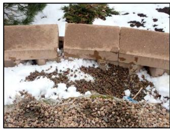
Figure 27: Closeup of soil subsidence behind CMU fascia wall and separation of capstone
