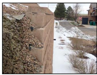
Figure 34: Undulations in Wall A where wall leans outward
