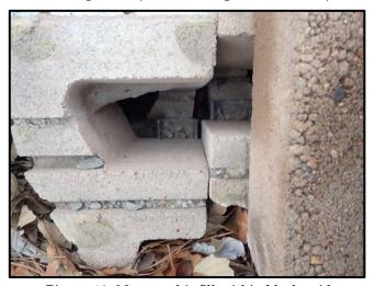
Figure 49: No gravel infill within block void
