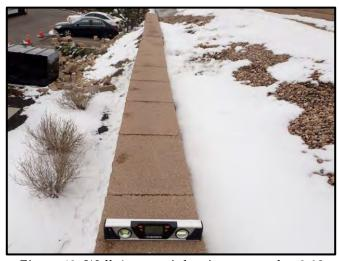
Figure 43: Wall A cap unit leaning outward at 3.9°
