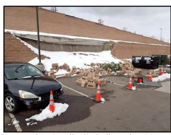
Figure 11: Overview of localized collapse of retaining wall
