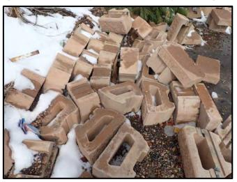
Figure 12: Scattered blocks and gravel fill
