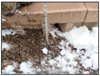
Figure 28: Approximately 12 inches of soil subsidence
