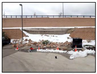
Figure 10: Overview of localized collapse of retaining wall
