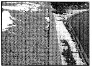
Figure 38: Undulations in Wall A where wall leans outward
