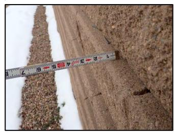
Figure 36: Proper batter of Wall B
