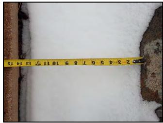
Figure 25: Space between shotcrete wall and back of cap unit approximately 15 inches
