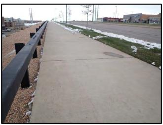
Figure 52: No signs of distress in concrete flatwork over retaining wall
