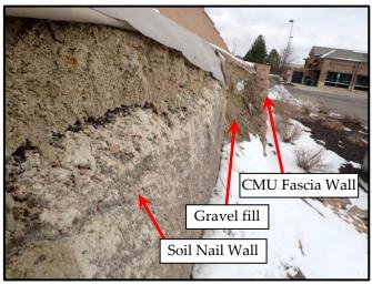
Figure 14: Lateral view of soil nail wall, gravel fill, and CMU fascia wall
