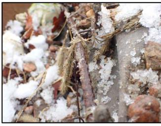
Figure 54: Exposed and corroded rebar in shotcrete soil nail wall; designed to have approximately 5 inches of cover
